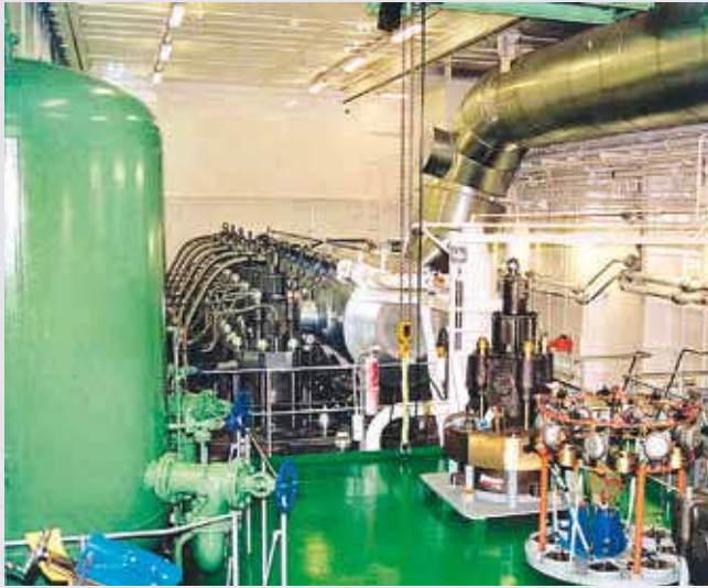
Ship engine cooling
